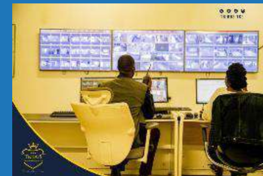
Security Operations Center
